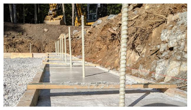
MST-BAR can eliminate the need for L bars in footing. Switch to dowels that can be wet set in after the concrete pour to save screed time and get a flatter footing.
